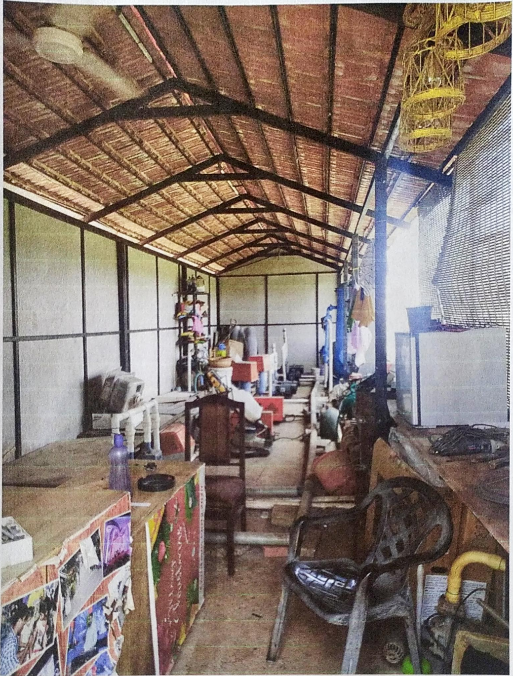
No. 5 : Internal area of STP with concrete flooring sy.no 55/3_Colva village. 164
